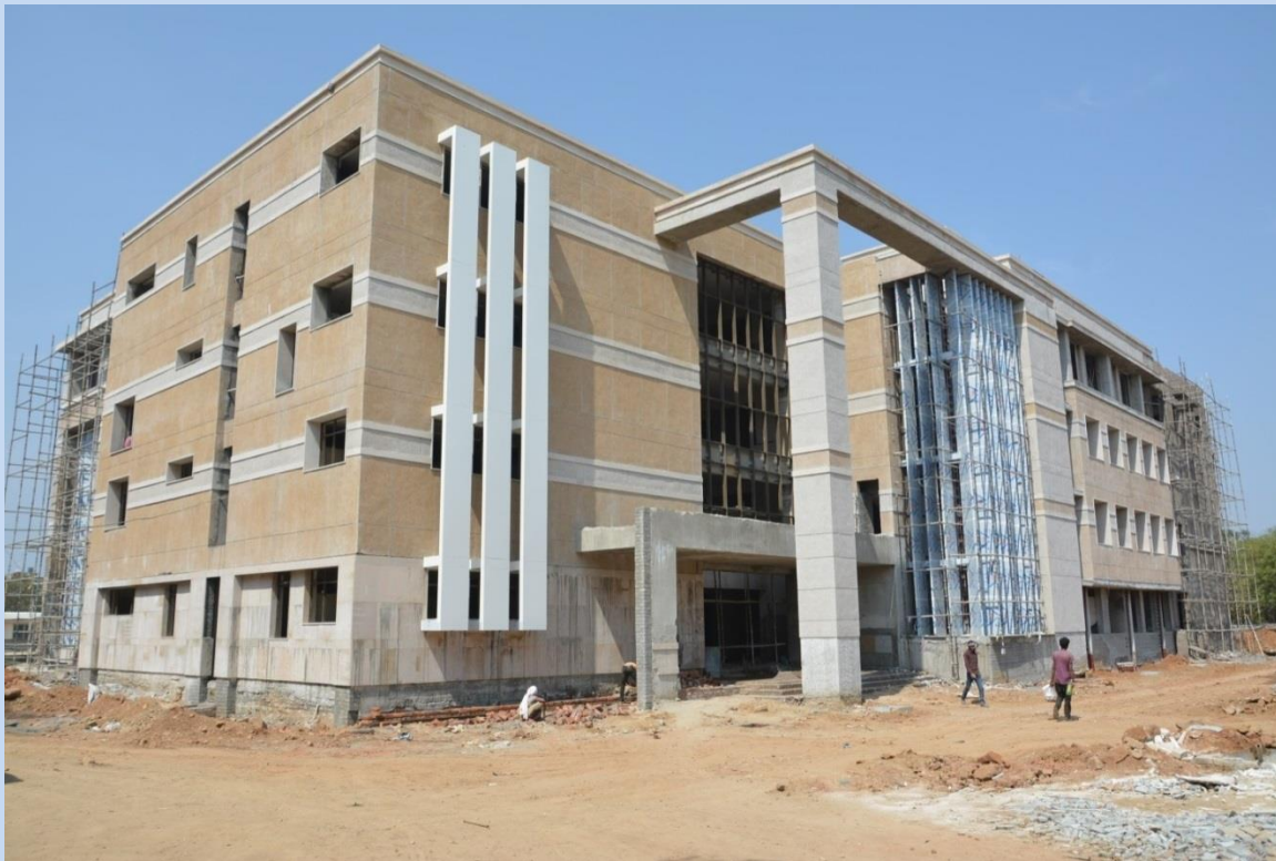
Upcoming New College Building
